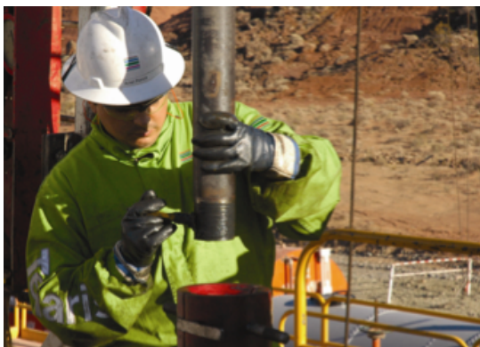
RUNNING COMPOUND APPLICATION.
